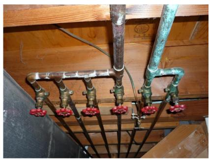
First identify the individually separated water supply lines going to each apartment. Turn off water and bleed pressure at a nearby faucet. Cut with appropriate pipe cutters (PEX, copper, etc.). Meter lay length is roughly 2.5-3.0" depending on preferred adapters based on your specific supply pipe material
