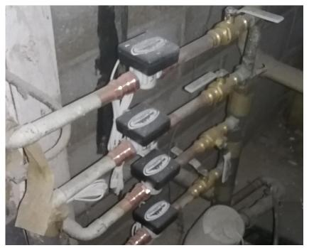
Finally, once installed, check for leaks and plug the power adapter into a nearby outlet. The meters are ready to go!
