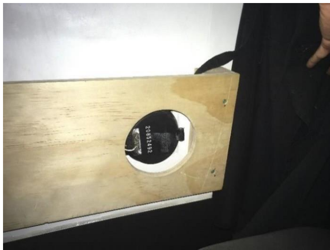
Figure 16. A water sub-meter, protected by a wooden case, installed in a bookkeeping space of a coffee shop.
