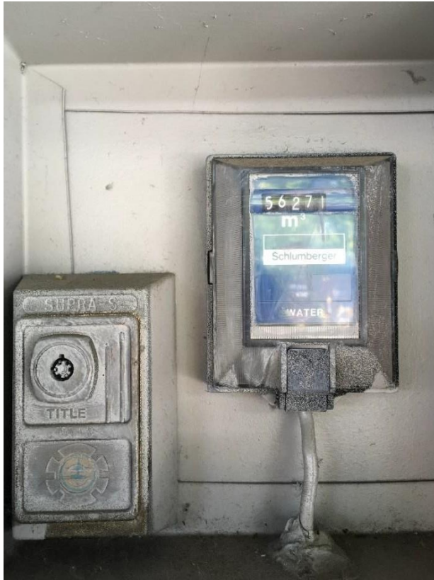
Figure 11. A manual reading water meter that measures the water use of a bakery on Granville Island.
